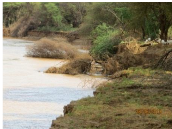
Plate 7-6: Severe bank erosion
