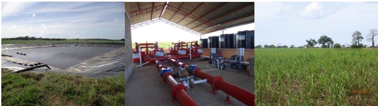
Plate 7-14: Kwale project using the three components of ground water and rainfall and water harvesting project
